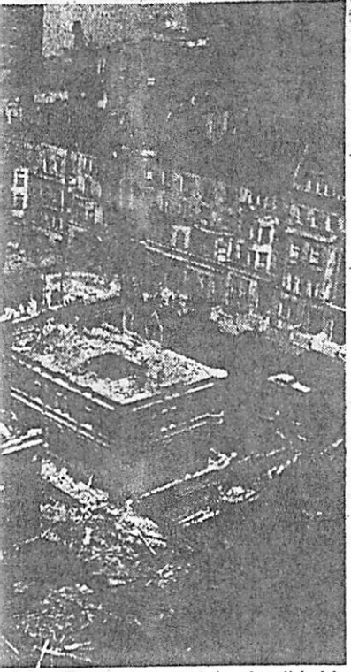
and Seventy-second Street, being demolished by apartment building.
